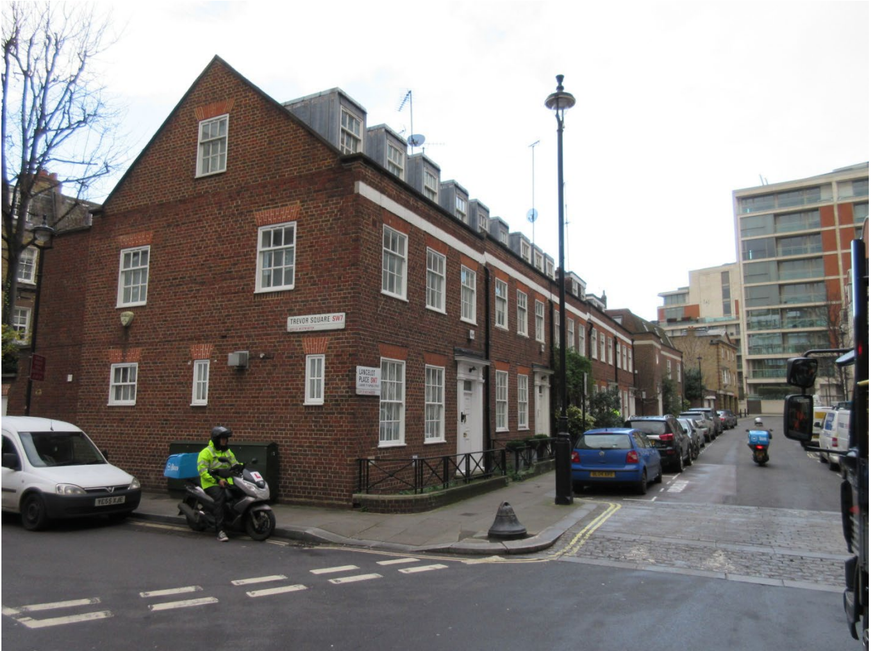
View of Application Site Prior to Demolition
